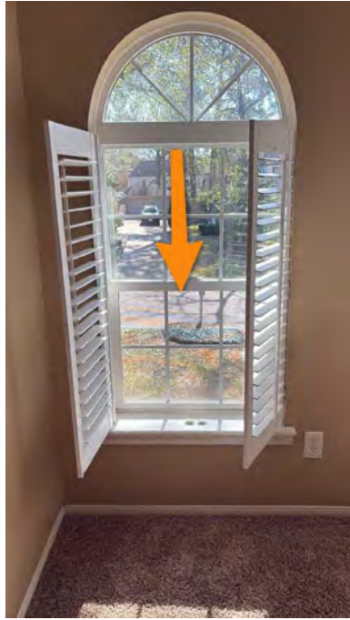
Primary left window- does not stay in up position
