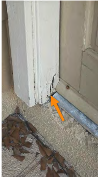
Garage door to back patio
