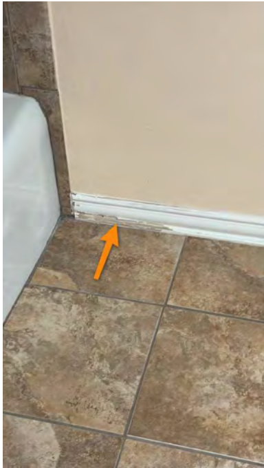
2nd floor bathroom
