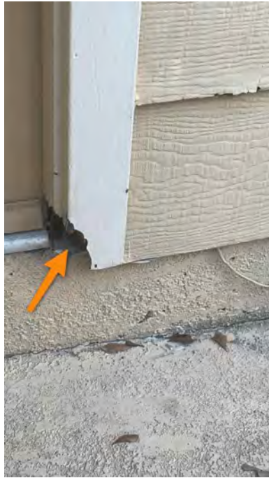
Garage door to back patio
