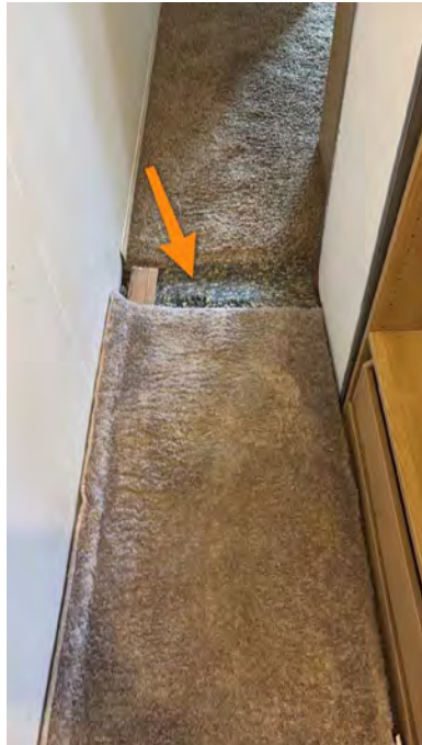
Primary / bedroom 2 closet
