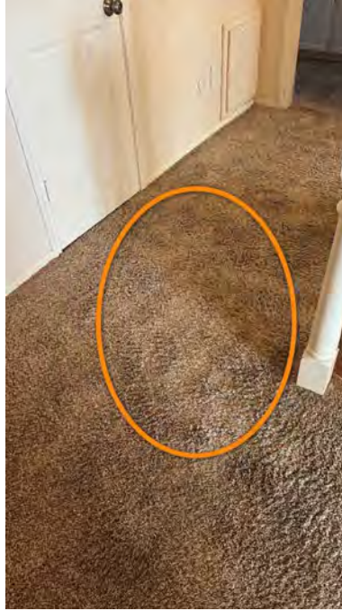
2nd floor hallway
