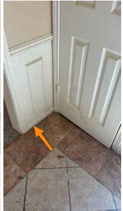
Front entry coat closet- uninstalled
