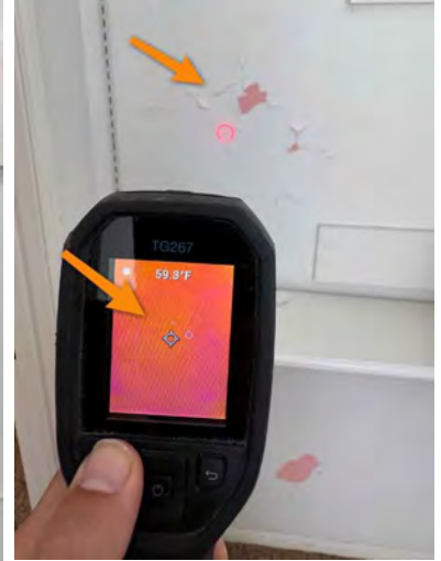
Bedroom 4 closet- Dry
