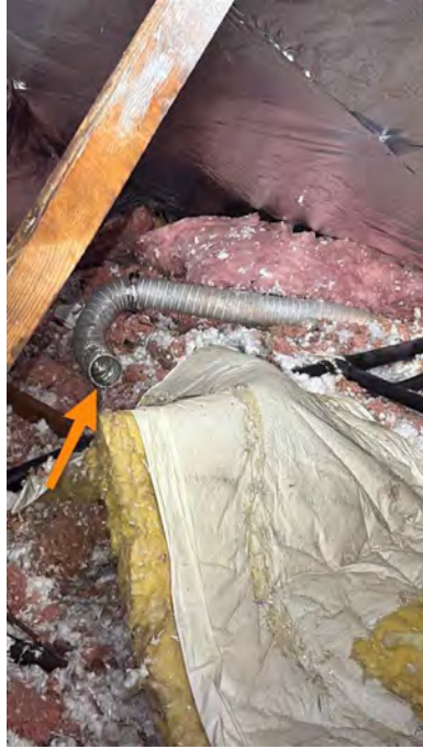
Venting into attic
