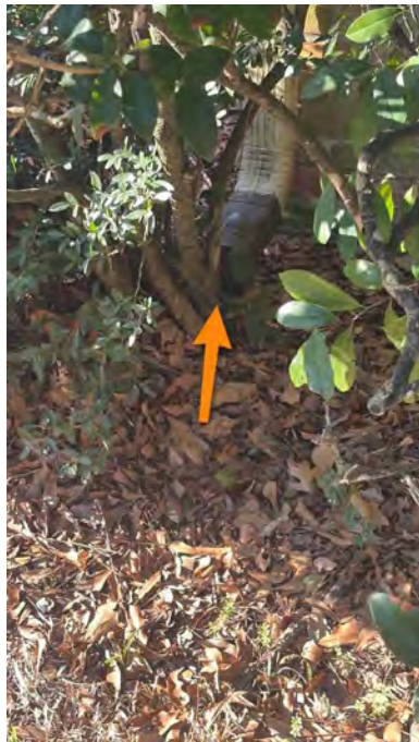
Right Side- extension does not not extend far enough
