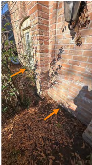
Front Left- grade to foundation clearance
