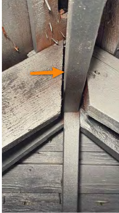
Garage attic access
