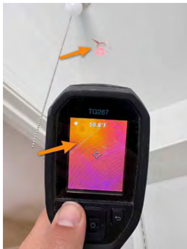
Bedroom 4 closet- dry
