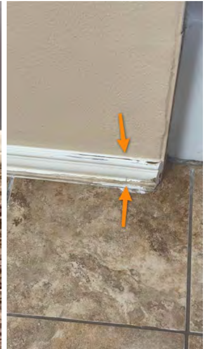
2nd floor bathroom
