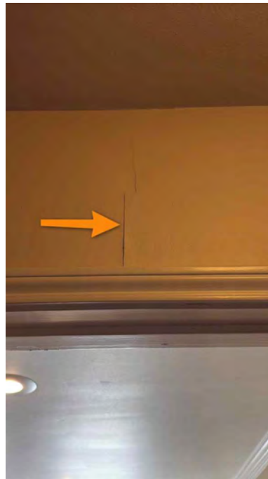
Above primary bedroom door
