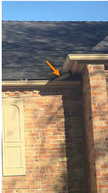
Front- upper to lower discharge
