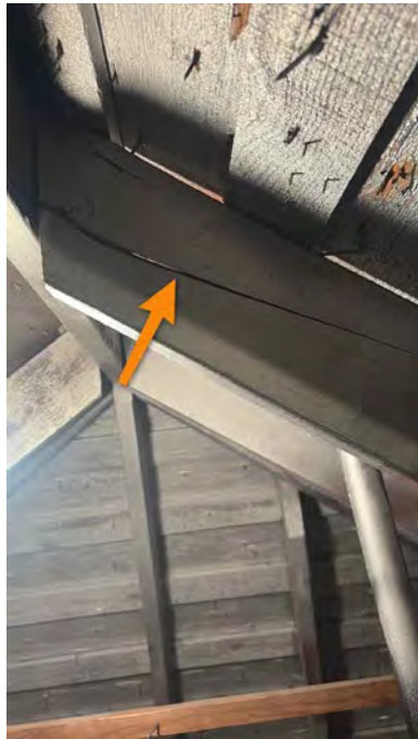
Garage attic access area
