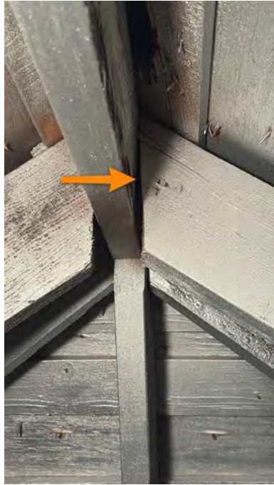
Garage attic access
