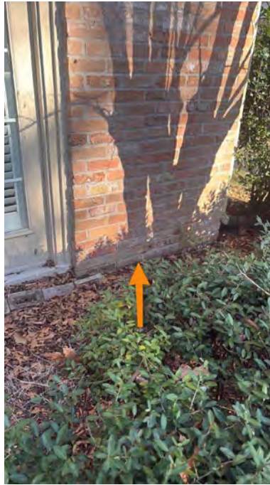
Front- grade to foundation clearance
