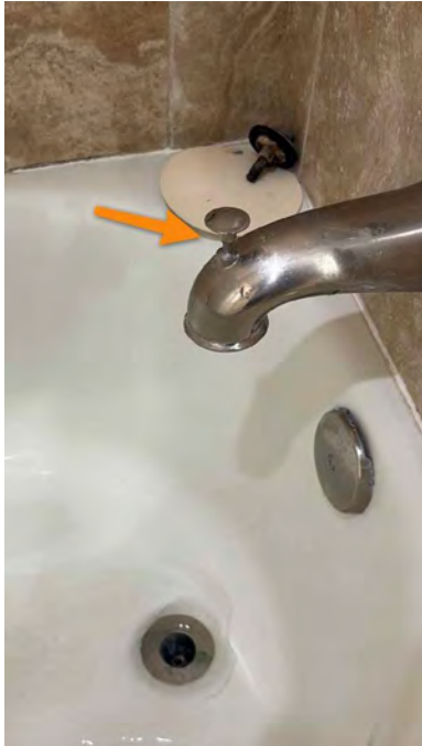
Primary tub- diverter stuck in shower mode
