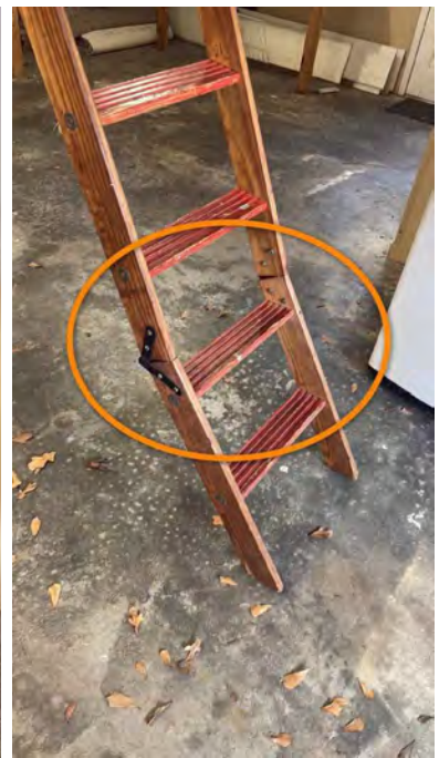
Garage attic- moose hardware
