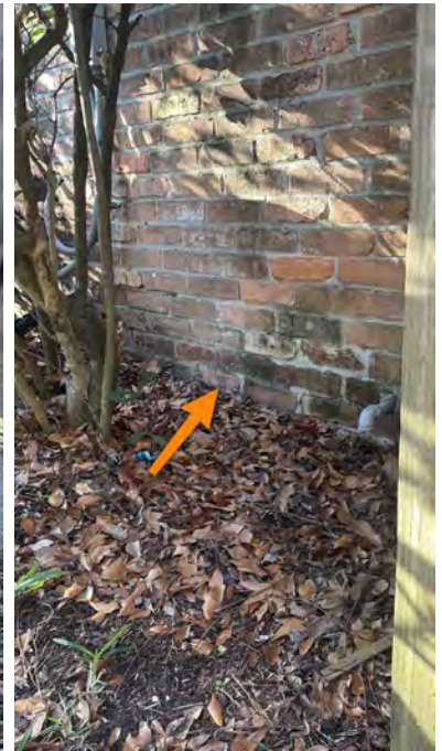
Right Side- grade to foundation clearance
