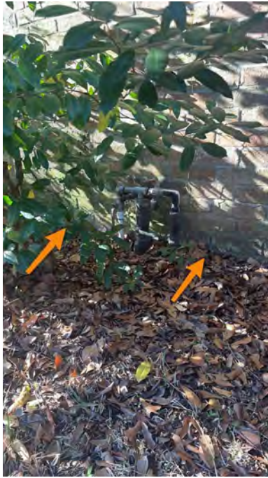
Right Side- grade to foundation clearance
