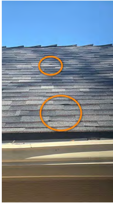
Above garage- lifted
