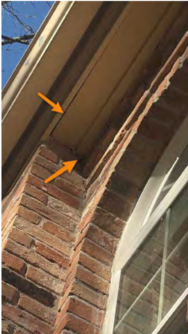
Front-opening and sealant
