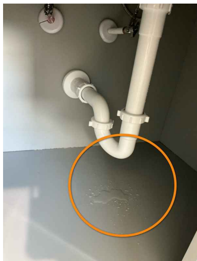
2nd Floor Bathroom
