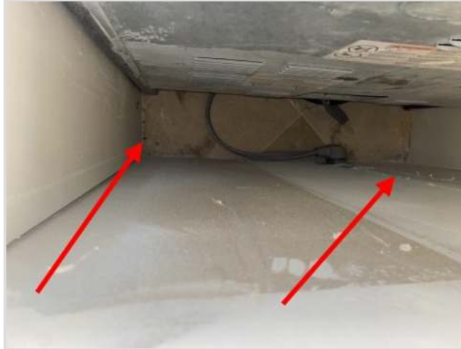
No anti-tip device installed
