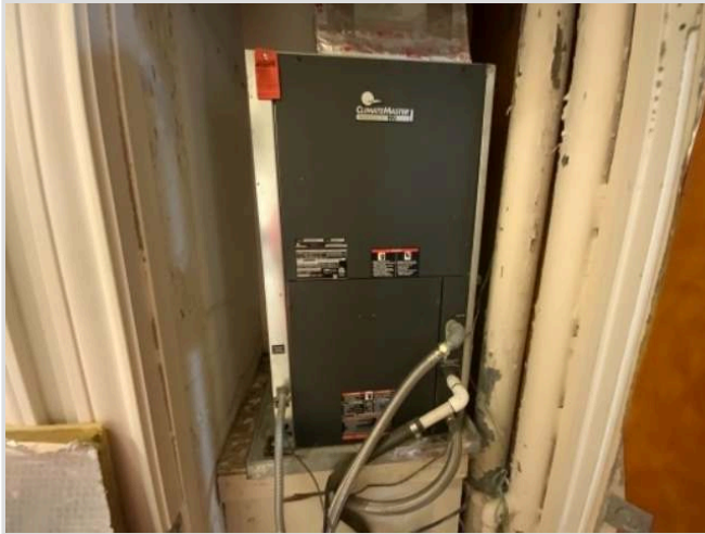
Geo-Thermal Heatpump
