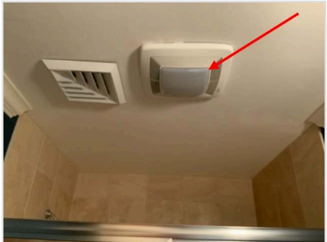
Would not illuminate (hall bathroom)
