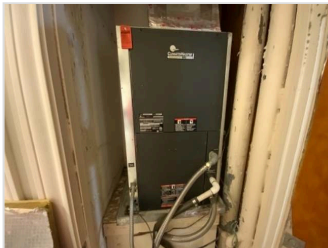
Geo-Thermal Heatpump
