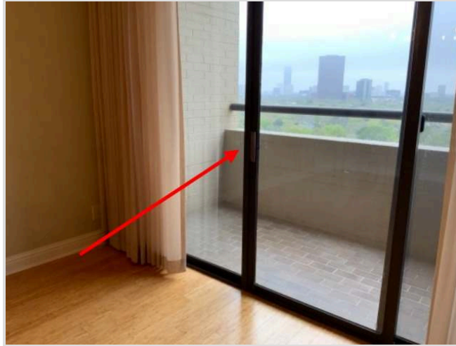
Latch damaged/broken
