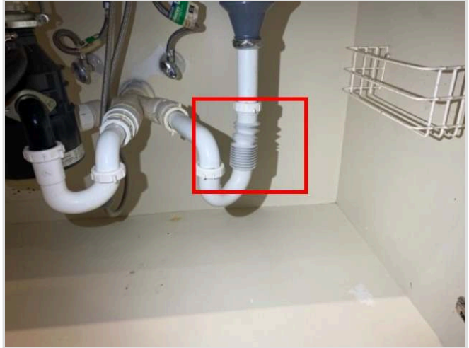
Improper material(kitchen sink)
