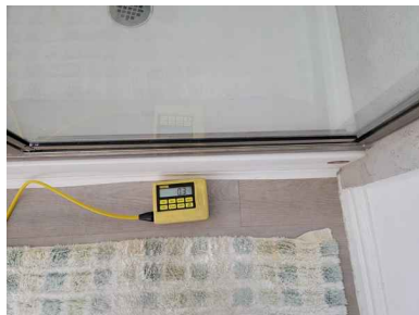
Right Side +0.3 Primary Bathroom
