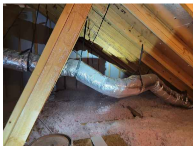
Rear Lower Attic
