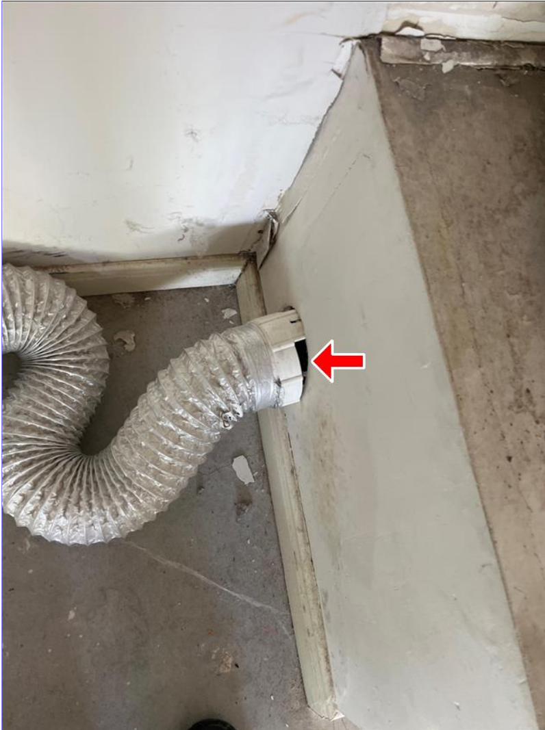
H. Item 1 (Picture) Garage
