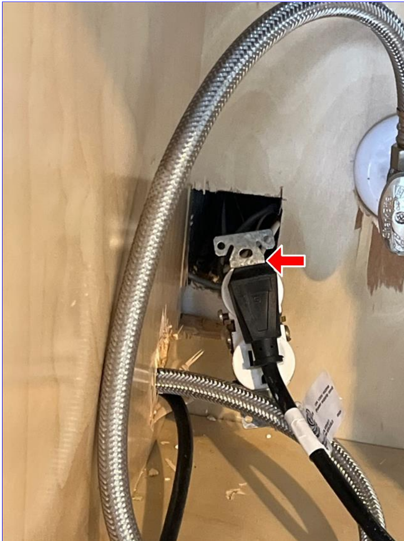
B. Item 5 (Picture) Kitchen sink cabinet
