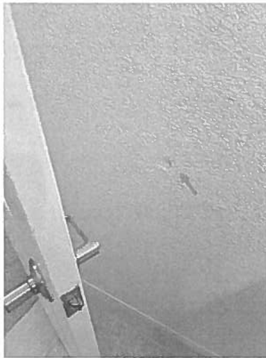
2nd Floor Bathroom
