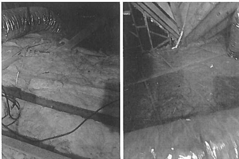
Approximate depth of insulation: 9.5 Inches (R-30) (2x10) -
