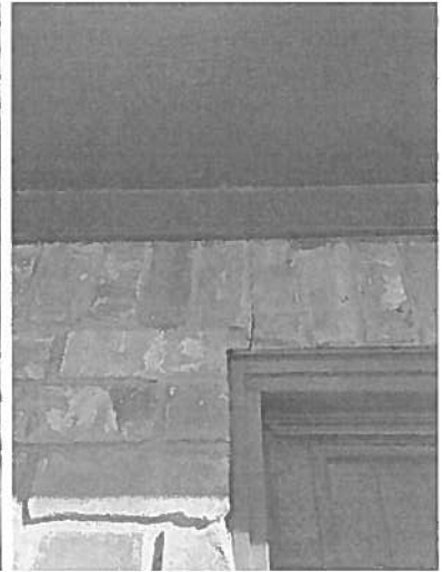
Garage Front Left
