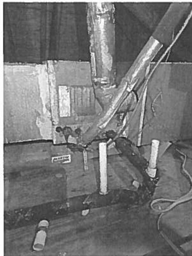
1st unit - measured temperature differential: Operable (15°F to 20°F) 1st Floor
