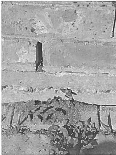
Garage Right Front
