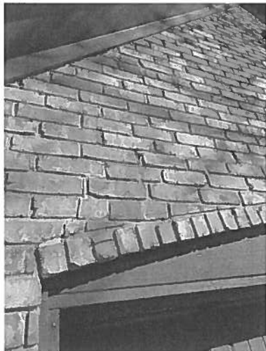
Garage Front Left
