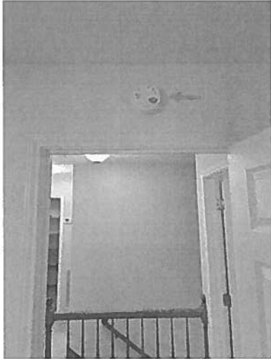
2nd Floor Back Left Bedroom
