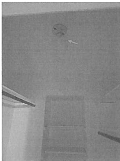
2nd Floor Back Left Bedroom Closet
