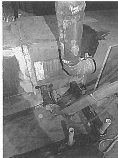
1st unit - measured temperature differential: Operable (15°F to 20°F) 1st Floor
