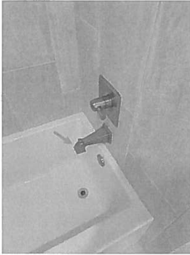
2nd Floor Bathroom
