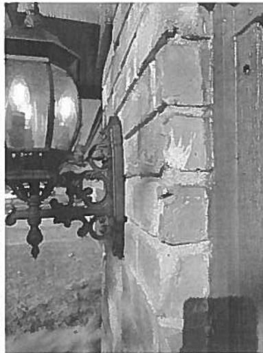
Garage Front Left
