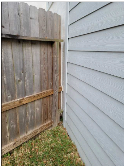
Wood fence in contact with wall..right side
