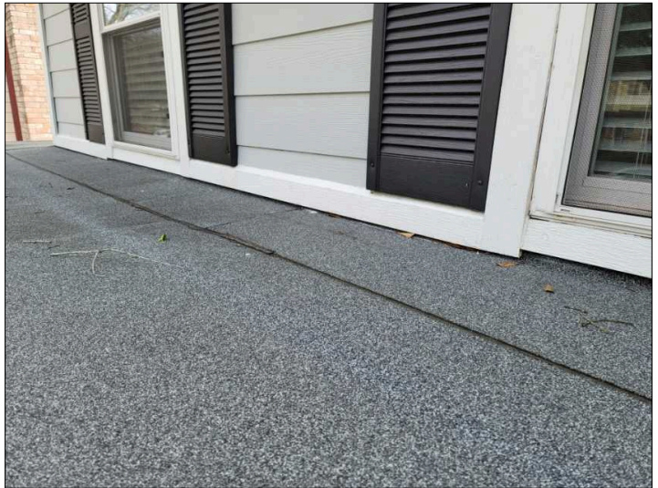
Roll roofing at low sloped section.. front over garage
