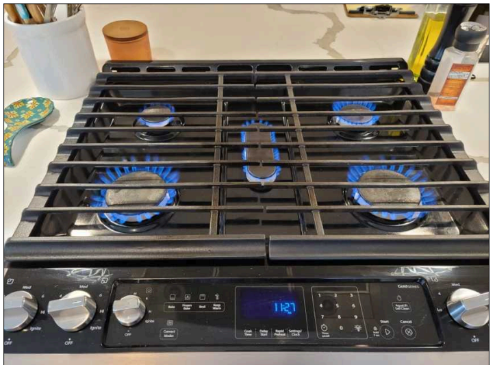
Gas range operational
