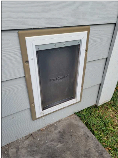
Pet door noted, installed at rear wall
