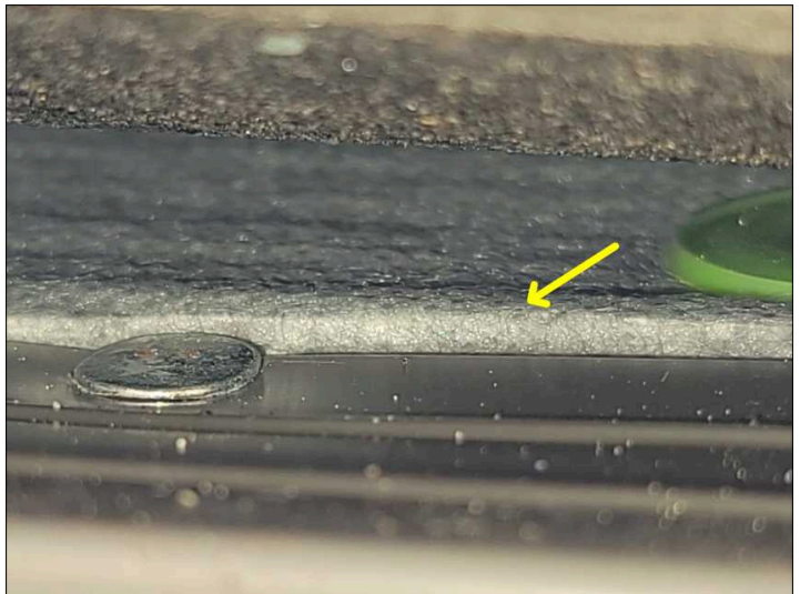
Roof felt underlayment should be on top of eave drip edge..front
