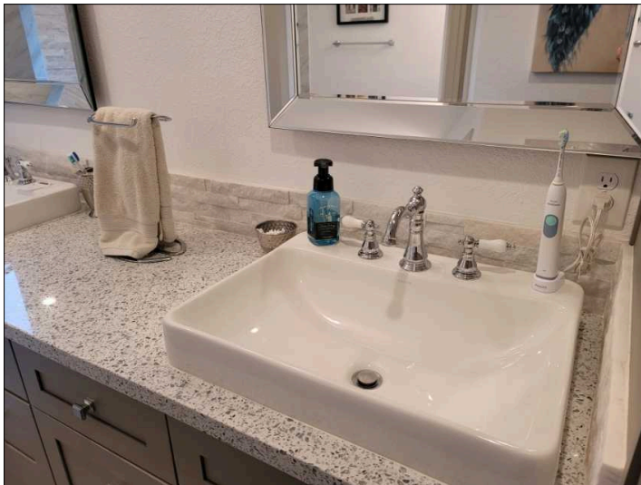
Lack of outlets, no GFCI protection..primary bathroom
