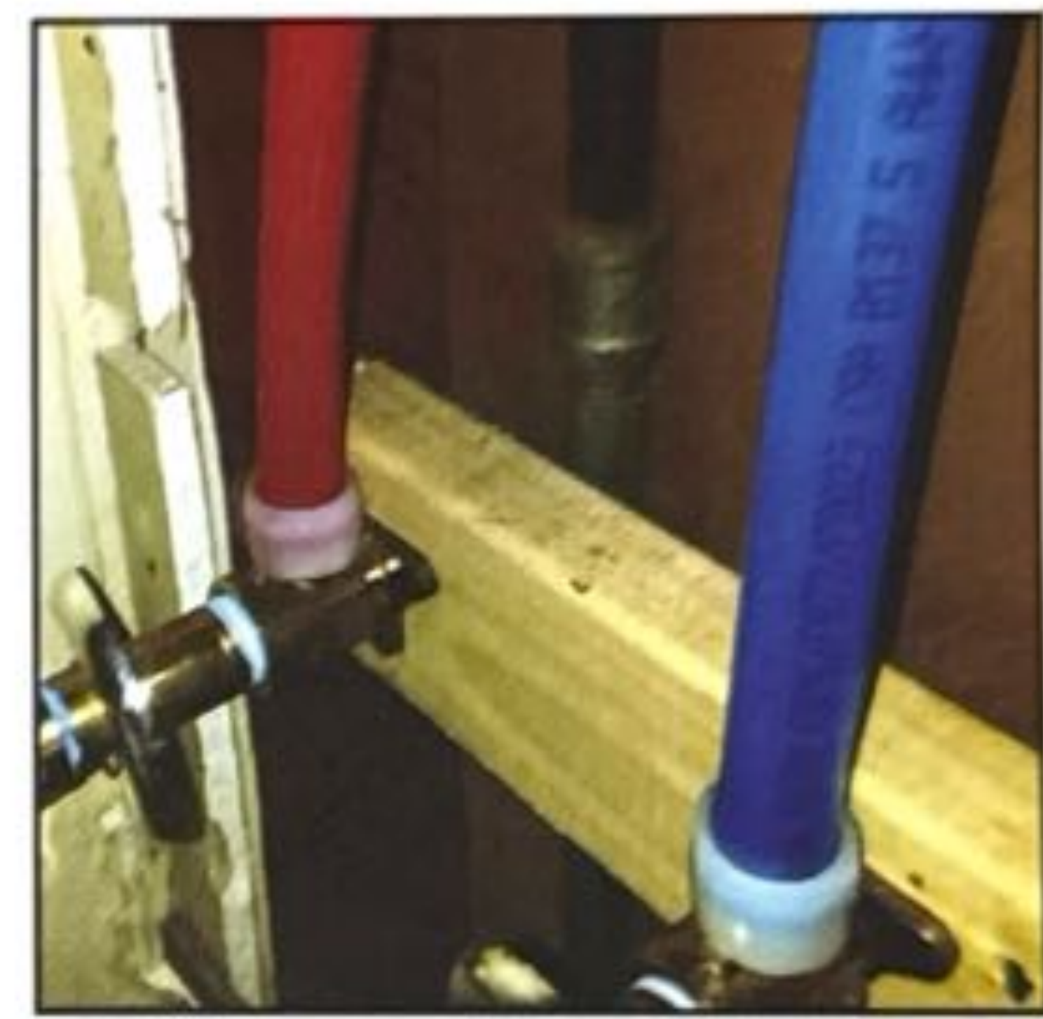
PEX PIPES RESISTANT TO FREEZE & CORROSION
