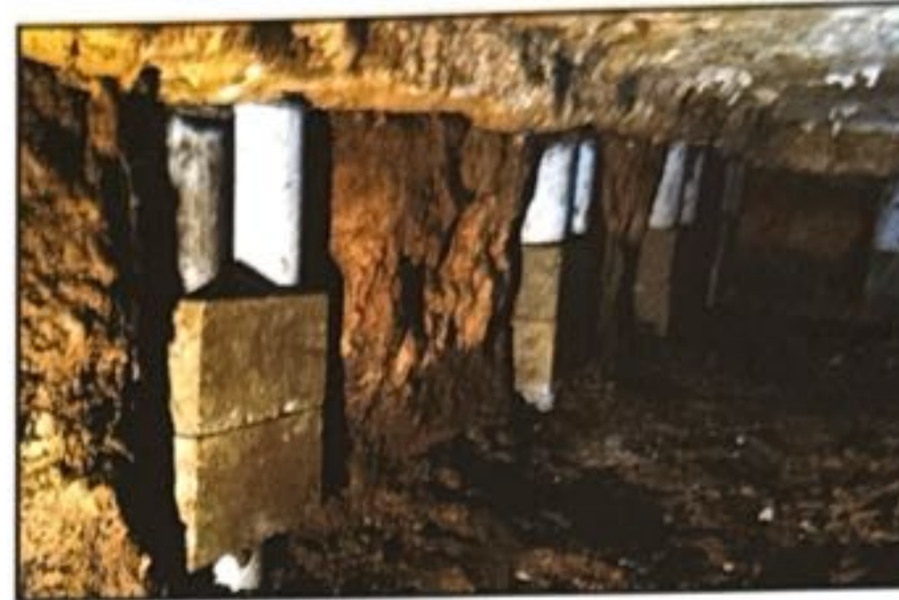
PILES INSTALLED FOUNDATION SUPPORTED
