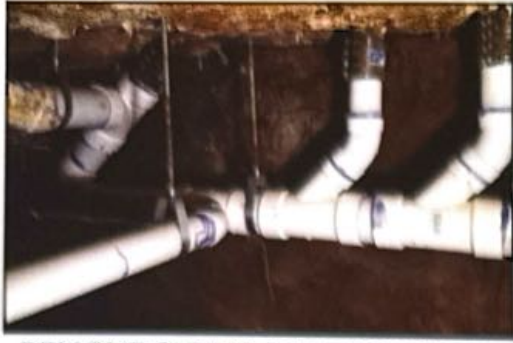
REMOVE & REPLACE CAST IRON WITH PVC
