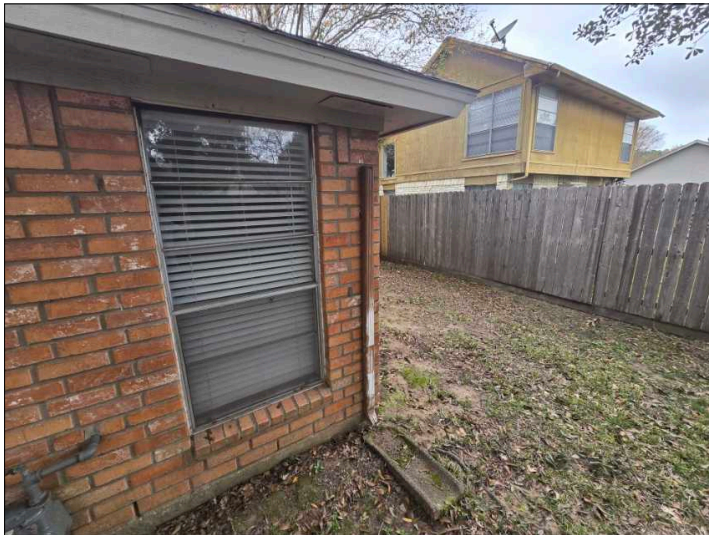
Removed gutters noted
