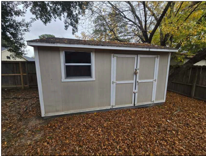
Building visually reviewed only.
