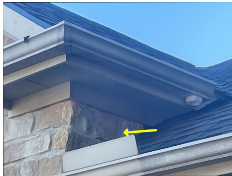
Missing flashing
