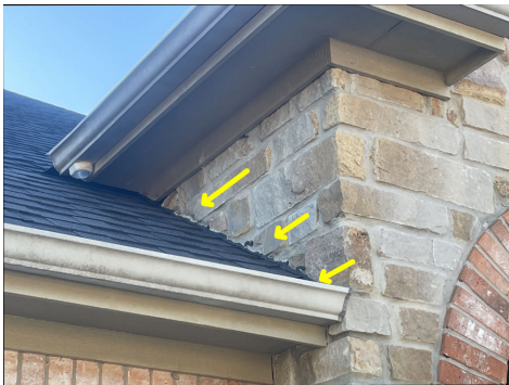
Missing flashing.
