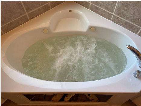
Spa tub operational
