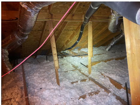
Missing insulation
