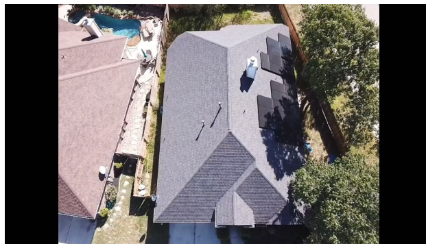
Drone photo of roof
