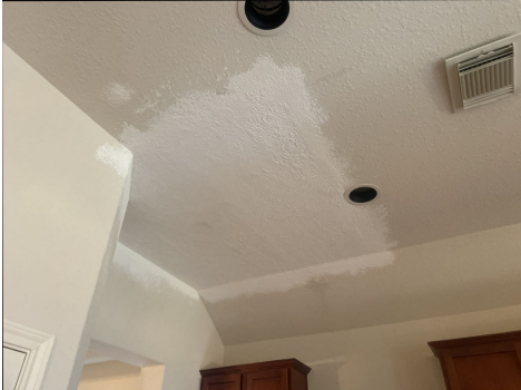
Repair in kitchen ceiling
