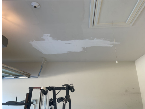
Repair in Garage ceiling.
