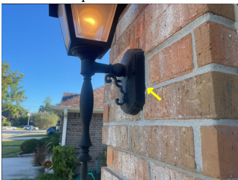
Seal exterior penetrations
